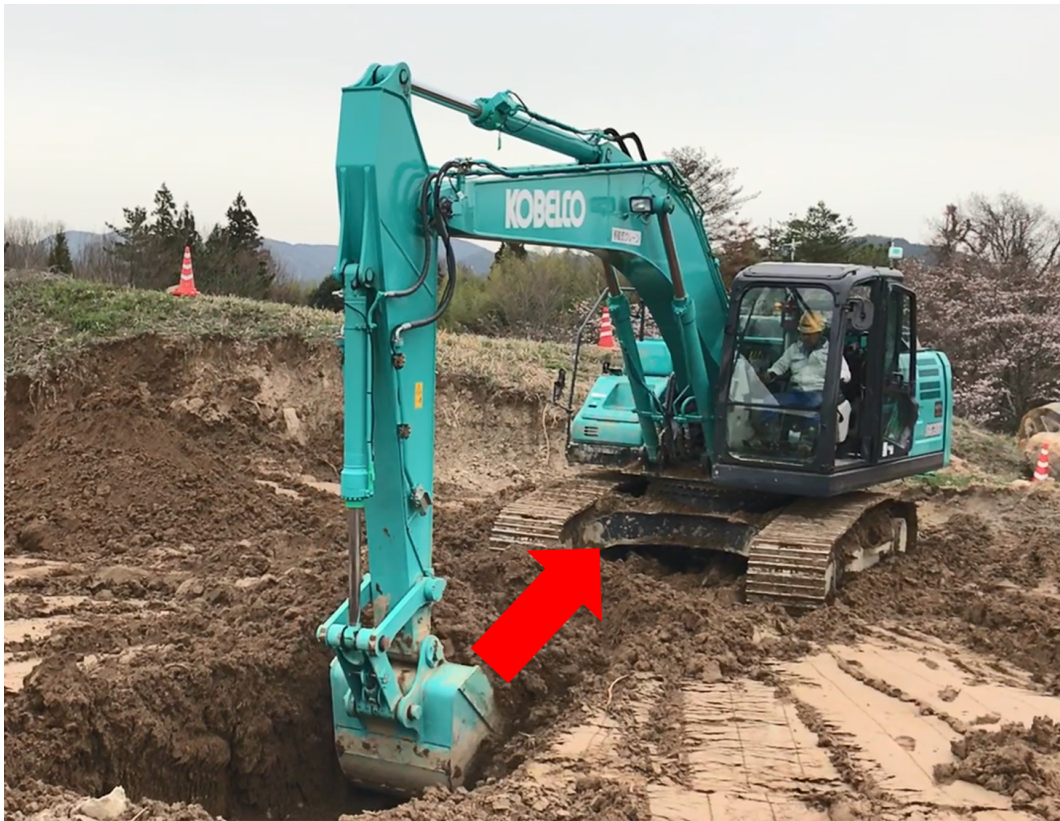
Fig. 2.1: Heavy load excavation.
