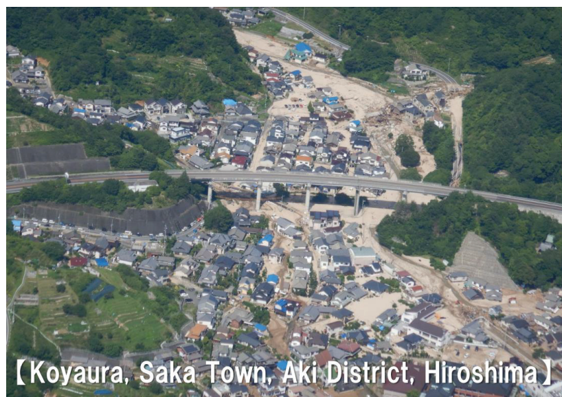
Figure 3-1. Road Damage in Hiroshima caused by the July 2018 Heavy Rain Disaster (MLIT, 2018)
