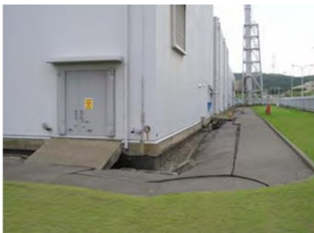
Fig. 2-4 Example of cracks occurring alongside nuclear power plant building due to soil settlement below the building<sup>2-41)</sup>
