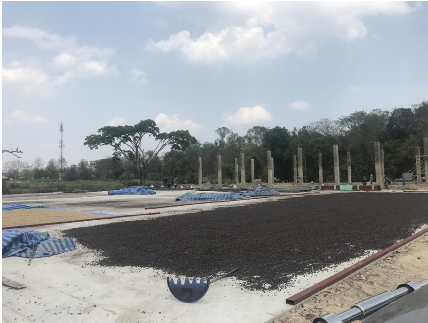
Figure 16 Mr. Kwan's coffee storage under construction
