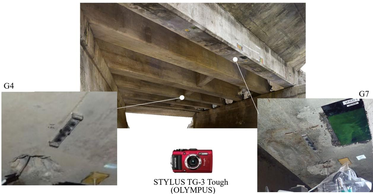
Fig. 7.3 Installation of strain visualization devices
