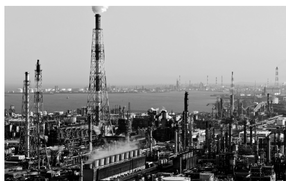
Fig.32. A view of an oil refinement and petrochemical complex ( Yokka-ichi ).
