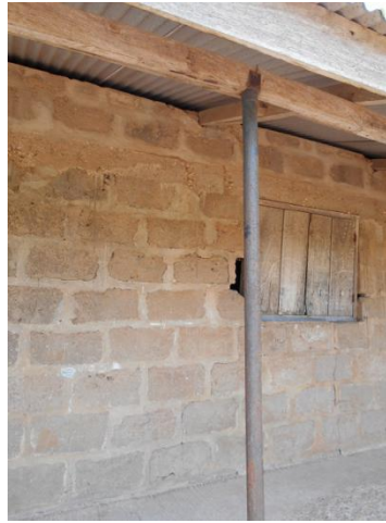
Figure 11. JHS block in danger of collapse due to lack of funds (School D) (left); Figure 12. JHS corridor buttressed with a temporal structure (School D) (right)
