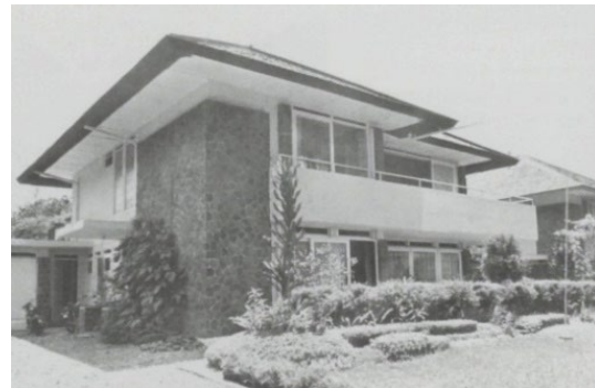
Fig2.15 Villa on Jalan Gunung Pager, Bandung by A.F. Aalbers (1939) 20)
