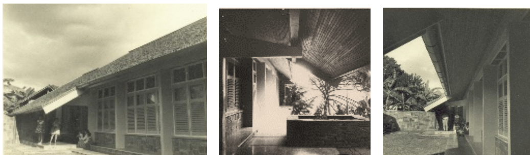
Photo4. 4 Silaban's house back veranda 7)
