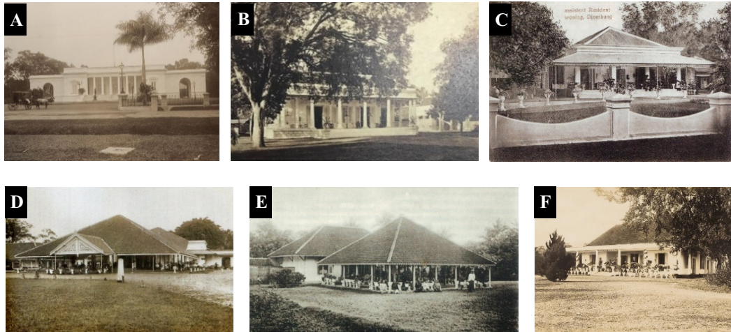
Fig3.10 The official house of the Dutch Indies government staffs 33-35) (A. Palace of the Governor-General at Batavia (1895, KITLV 81596), 35) B. House of the resident of Batavia, 33) C. House of the assistant resident of Djombang (1916), 34) D. House and pendopo of the regents of Wonosobo (1925), 34) E. House and pendopo of the wedana of Cheribon (1910), 34) F. House of the administrateur of the sugar factory of Paroengdjaja, Madjelengka (circa 1890-1895, KITLV 55912) 35)
