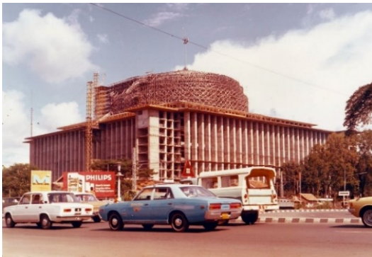
Fig2.71 Istiqlal Mosque's construction project (1973) 7)
