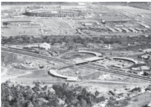
Fig2.27 Semanggi bridge and Senayan stadium complex (1962) 28)
