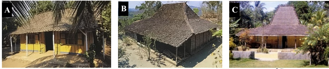
Fig3.7 Front veranda ( emperan ) in traditional Javanese houses 24) (A. Kampung -style house, B. Limasan -style house, C. Joglo -style house)
