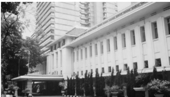
Fig2.8 Batavian Petroleum Company office by Thomas Nix (1937) 11)
