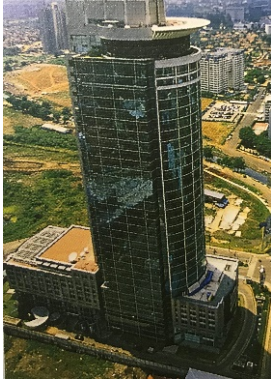
Fig2.67 Emporium Tower, Kuningan, Jakarta 6)
