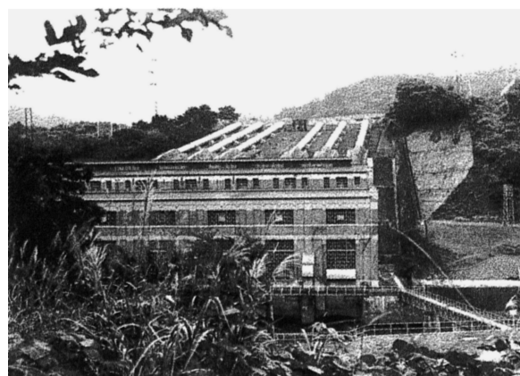
Fig.22, The First Inawashiro Hydroelectric Power Plant under the construction and after the completion.
