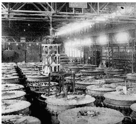
Fig.24, The calcium cyanamide reactors in Minamata factory of Nihon Chisso-Hiryō Kabushiki-Kaisha
