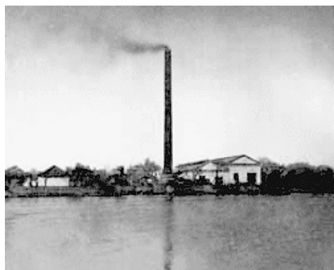
Fig.21, Asakusa Power station
