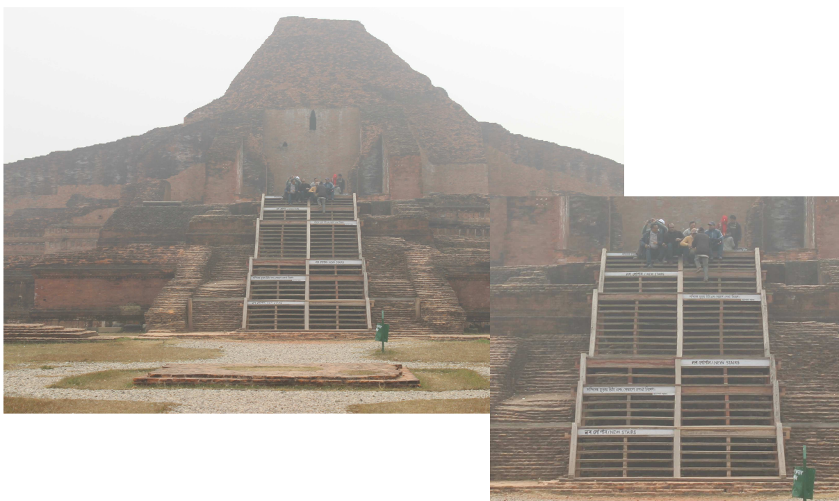
Figure 82 Iron-framed wooden staircase installed by SATIDP in the Central Shrine of Paharpur
