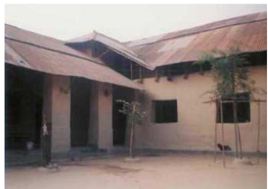
Figure 81 Mud Architecture in Mahasthangarh Region (Das et al. 2007)
