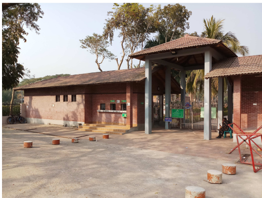
Figure 78 SATIDP -installed gateway at Bagerhat
