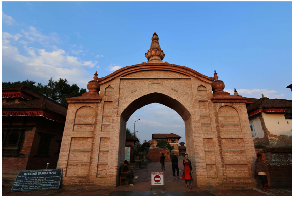
Figure 56 Rebuilt Central Gateway of Bhaktapur Durbar Square by following the Mollar Architectural Style after the destruction by the earthquake in 2015
