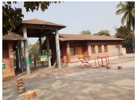
Figure 79 SATIDP -installed Gateway at Paharpur
