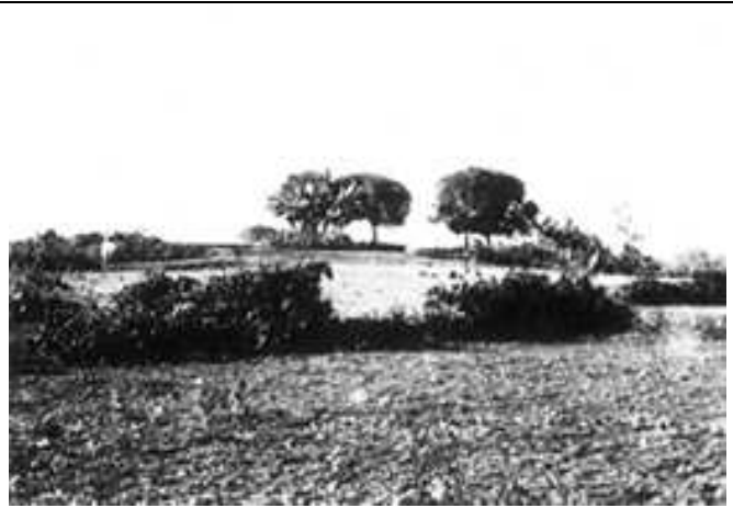
Figure 9 Bairagir Bhita, Mahasthangarh
