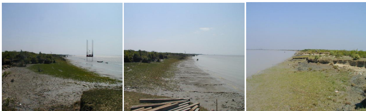
Photo - 5.2 Conditions of shoreline of Yangon River at Thilawa
