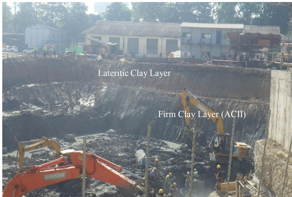
Photo - 4.3 Conditions of underground at Central sub-area in Yangon
