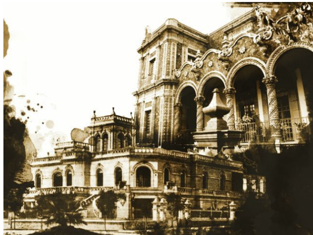
Fig. 8 Building of eclectic style built during the Porfiriato in Guadalajara, Jalisco, Mexico between 1895 - 1911 (López García, 2010).
