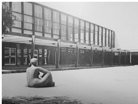
Fig. 44 Glassed façade of NSA (INBA, 1986)
