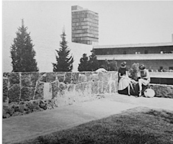
Fig. 45 Open area inside to NSA (INBA, 1986)
