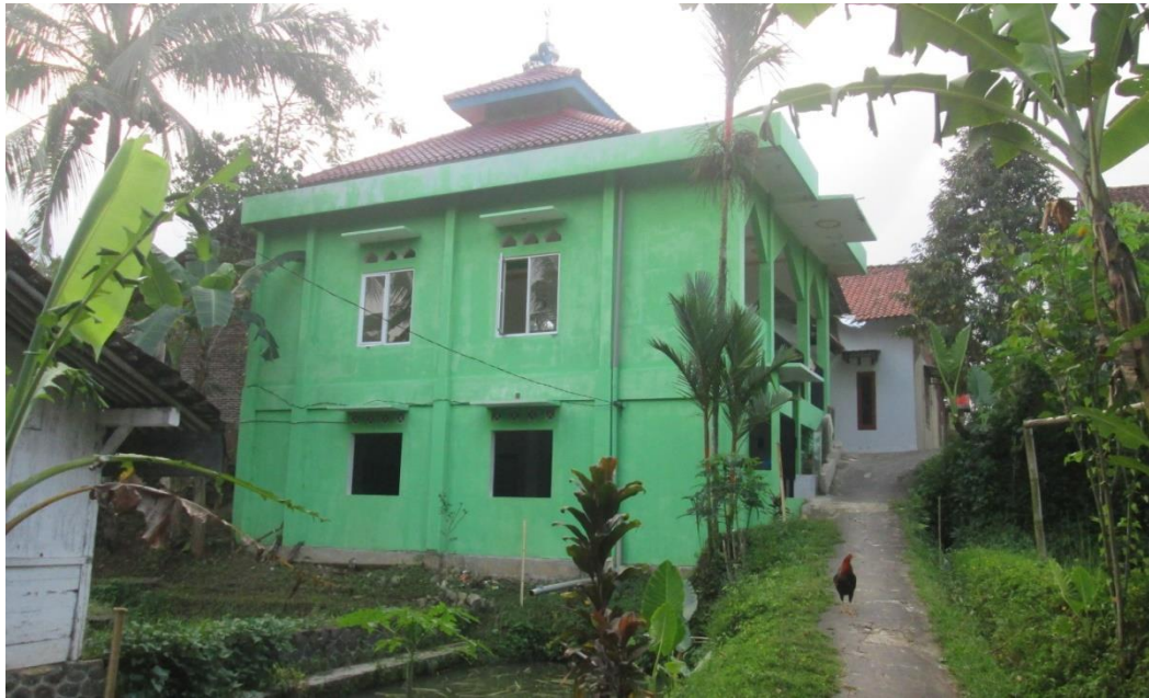
Fig 5.1 Baitul Falah Qur'anic School building (first floor) in Luwung village
