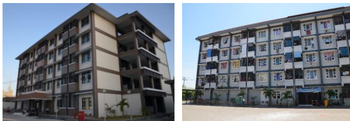
Figure 3.2. Views of new public apartment
