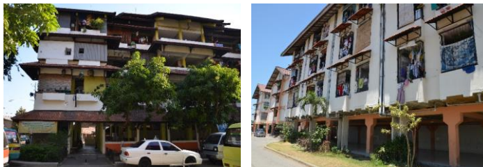
Figure 3.1. Views of old public apartments.
