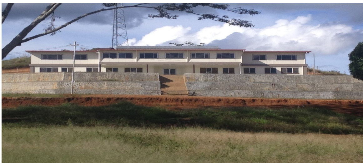
Figure 9 Ungai-Bena new district office under construction (Source: Author)
