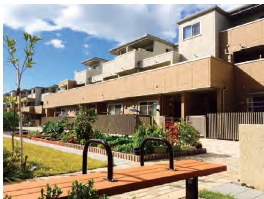
Figure 12 Ishinomaki City Public Restoration Housing, Shinhebita Area
