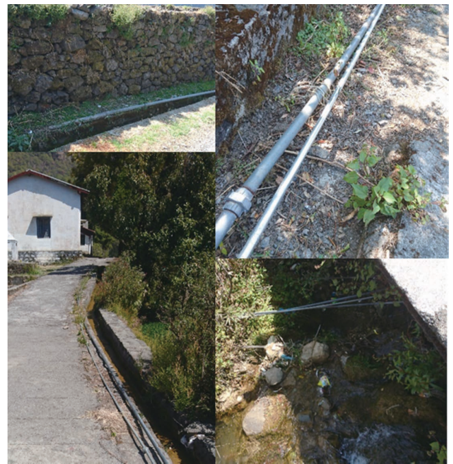
Picture 1. Pipelines and irrigation canals seen throughout the village Source: Ohnishi, March 2017
