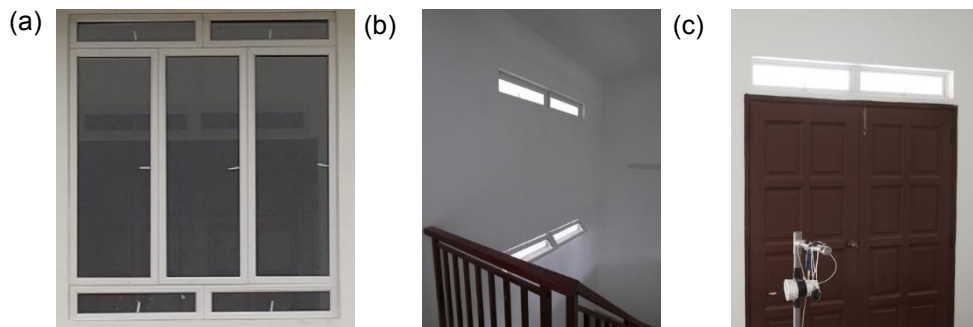
Figure 4.4. Position of slit windows (a) Upper and lower part of the main windows; (b) Upper and lower parts of partition walls; and (c) Upper part of door
