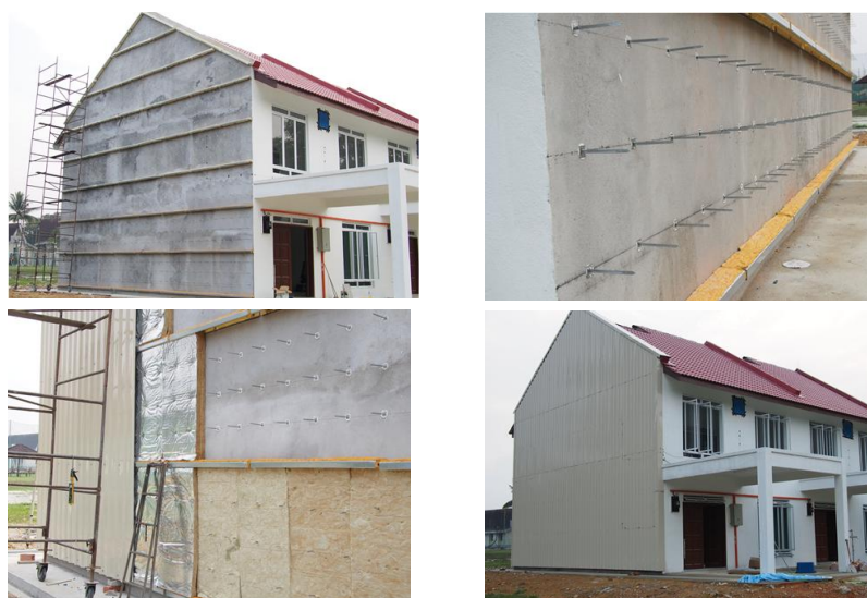
Figure 4.7. The installation process of the end wall insulation.
