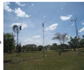
Wind Mill & Monitoring Equipment
