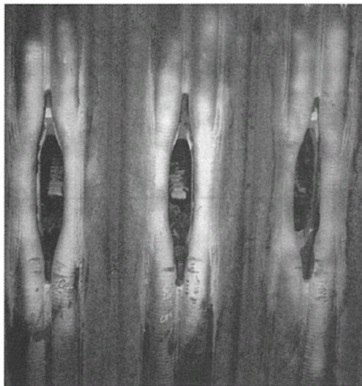
Fig.1.18 Primary air port openings fabricated from alloy 625 overlay tubes have been in service since 1999. No cracking or corrosion has been observed. The photo was taken after liquid dye penetrant testing
