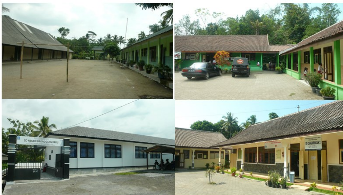
Figure 5.1 Typical school buildings in the research site
