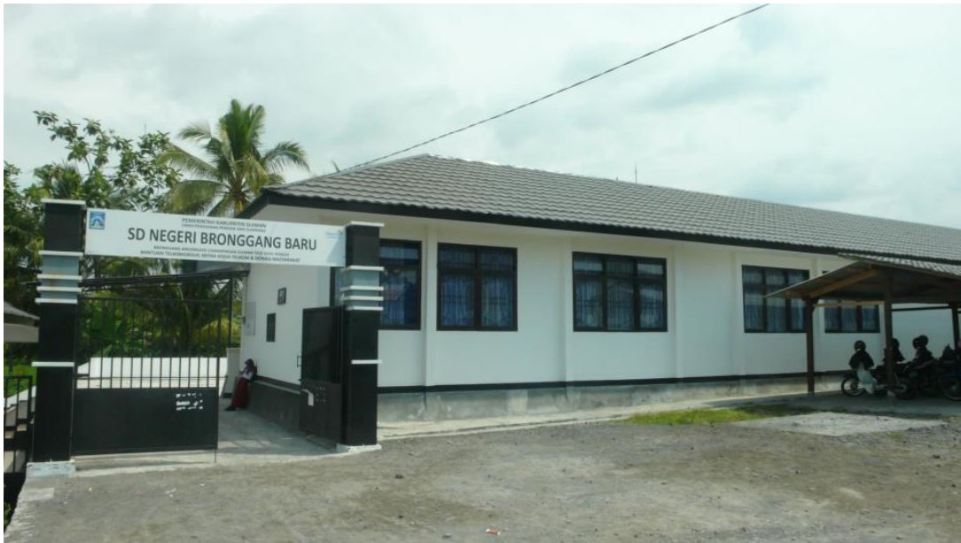
Figure 6.1 Renovated school building by Telkom in Cangkringan district
