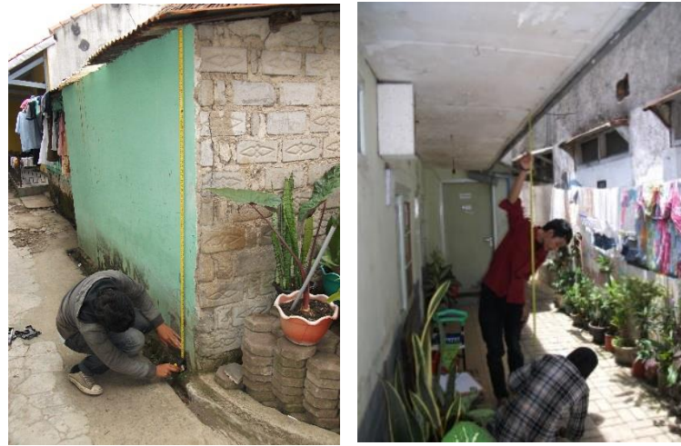
Fig. 4.6 On-site measurements; Building material inventory
