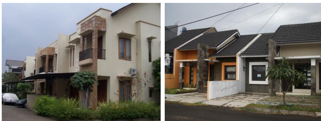
Figure 3.6 Planned houses in Jakarta city
