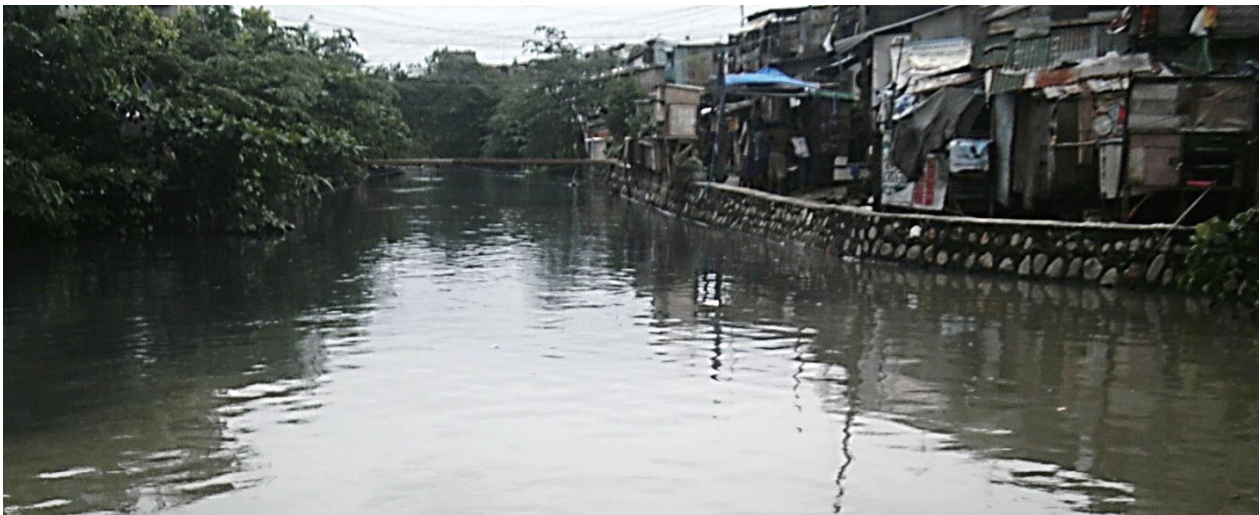
Figure 10. Section of Catmon Creek wall at Letre Canal Confluence on 2 Aug. 2012 (Photo credit: Malabon City, 2012)
