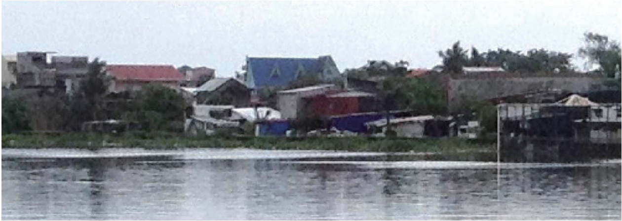
Figure 5. Functional river wall upstream in Tonsuya (Photo credit: James Tyree)
