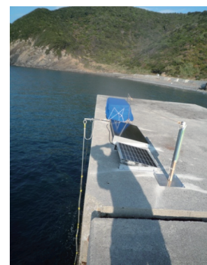
CATS picture on Fukudomari Breakwater (Saiki, Oita)
