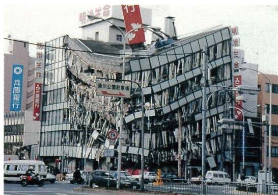
Collapsed due to torsional vibration (Kobe 1995)
