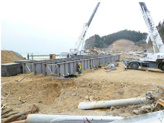
(a) Site of temporary construction
