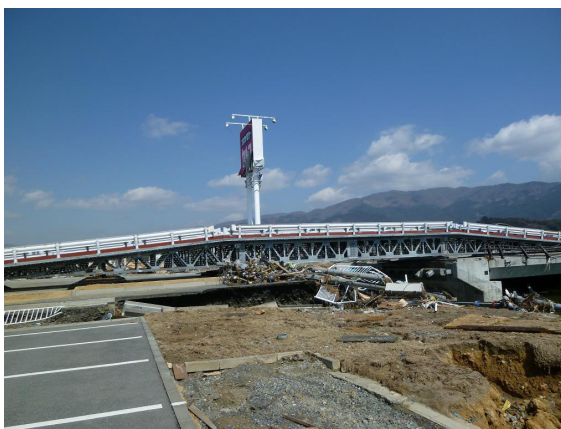
(b) Another completed reconstruction
