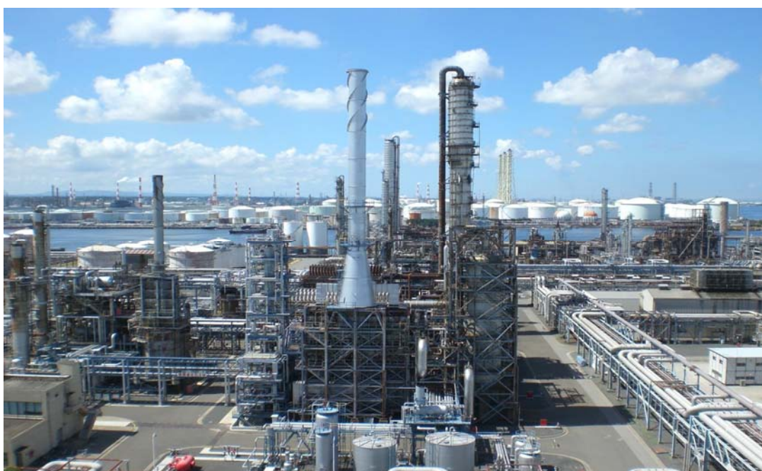
Fig.1.1.1 Appearance of Refinery and petrochemical industries
