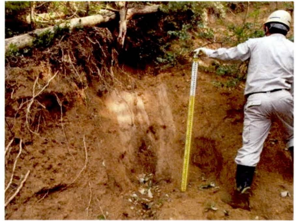
写真-5.3 崩壊源頭部のパイピング湧水 Photo 5.3 Piping-spring water at the head part of slope failure (図-5.22 中の②)
