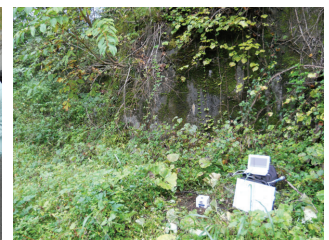
Kurikoma dam (Down stream bedrock)
