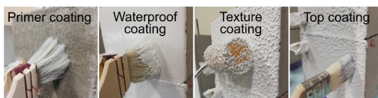
Figure 3–23 Photos of waterproof coating process.
