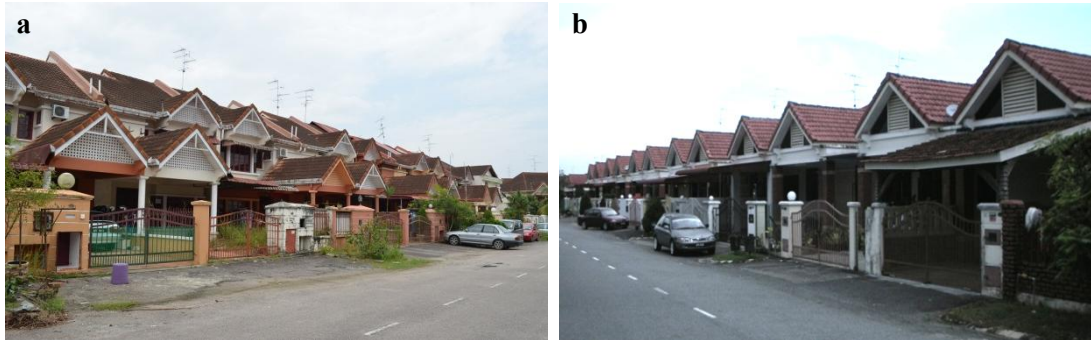
Figure 4.1. Typical modern terraced houses in Malaysia. (a) Double-storey; (b) Single-storey.
